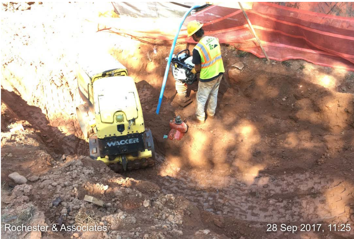
Photo 2: Both water main valves (#1 pictured above) are installed and require backfill and compaction.
