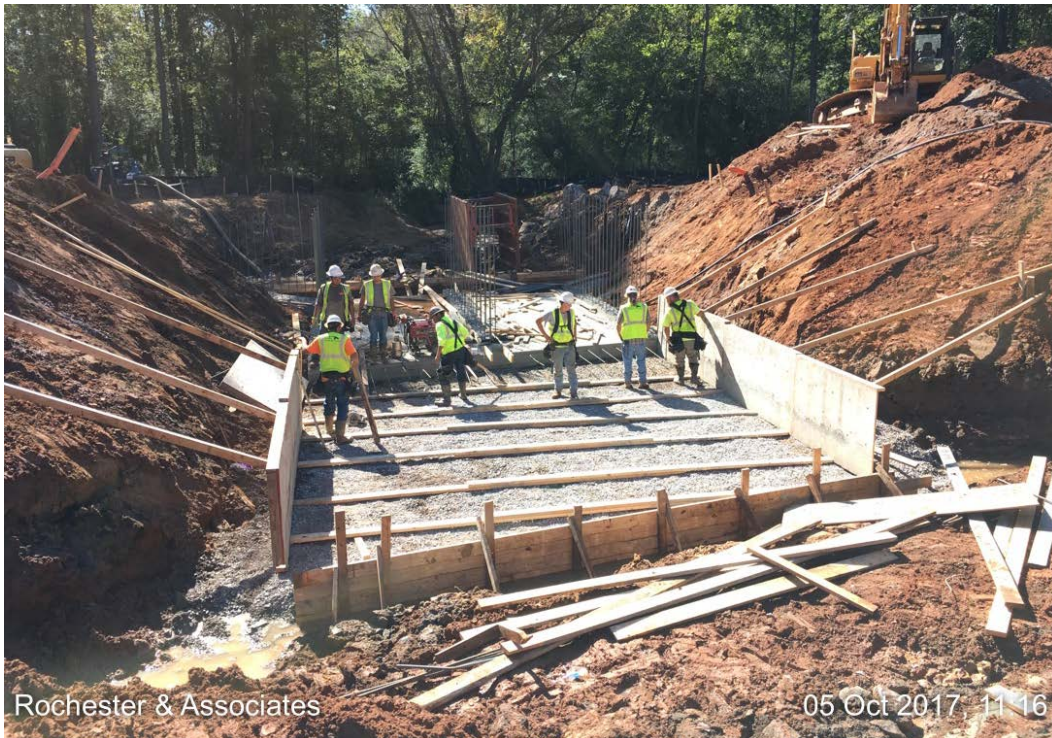
Photo 2: The bottom plate and wingwall footer construction is complete for first half of new culvert. Concrete forms and rebar are being placed for second half of culvert.
