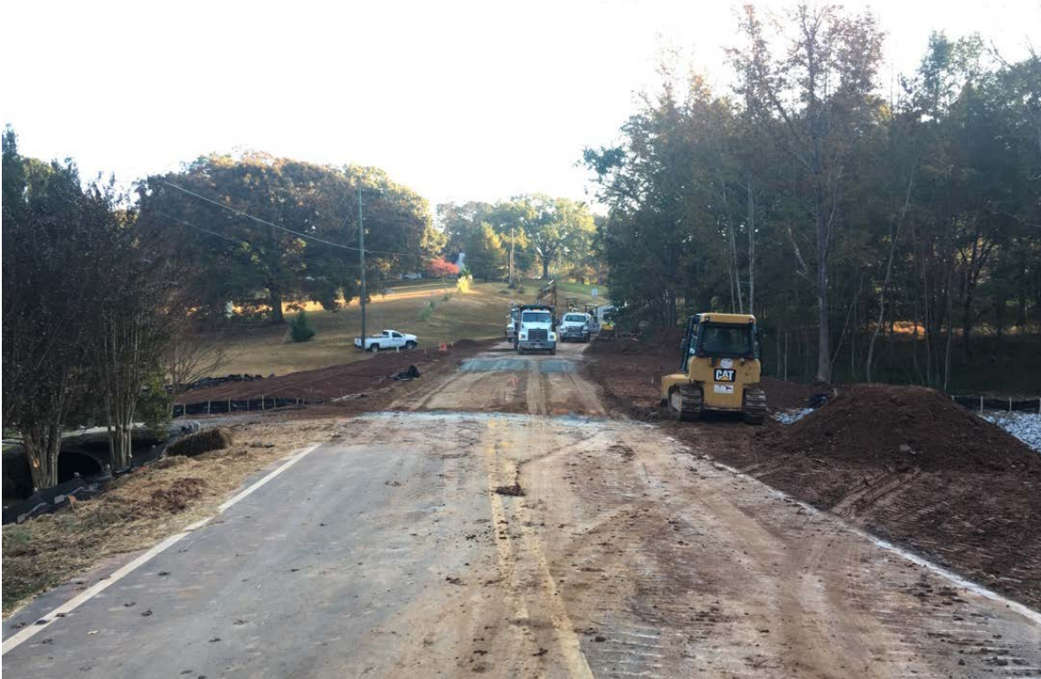
Photo 1: Roadway is being prepped for future paving.
