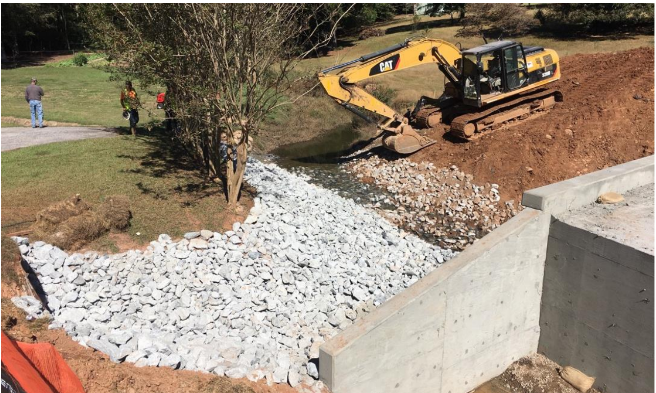
Photo 2: North of culvert: Grading, filter fabric and rock is in progress. (10/19/2017)
