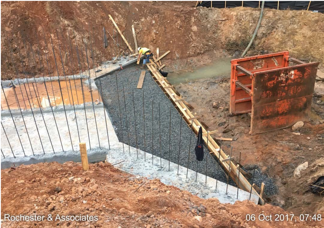
Photo 2: Gravel is placed in the apron area of the culvert.
