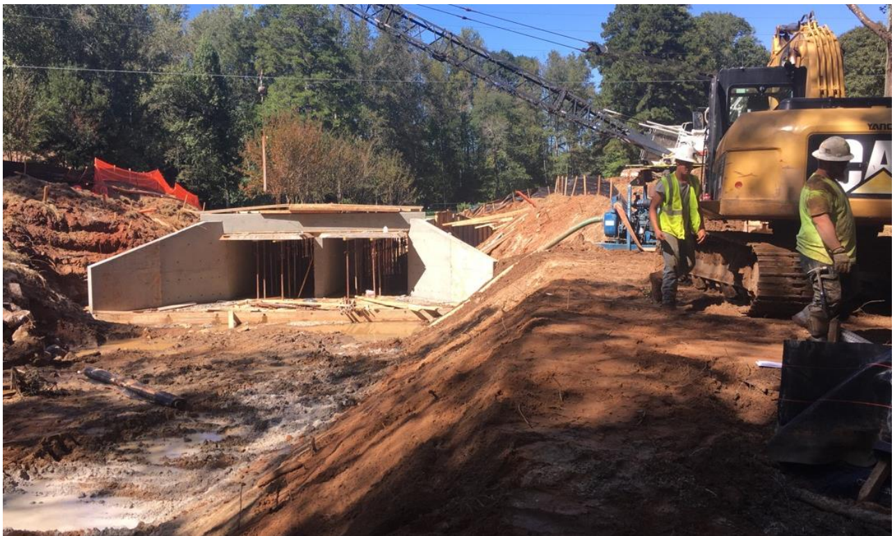
Photo 2: South of culvert: Grading has been initiated.
