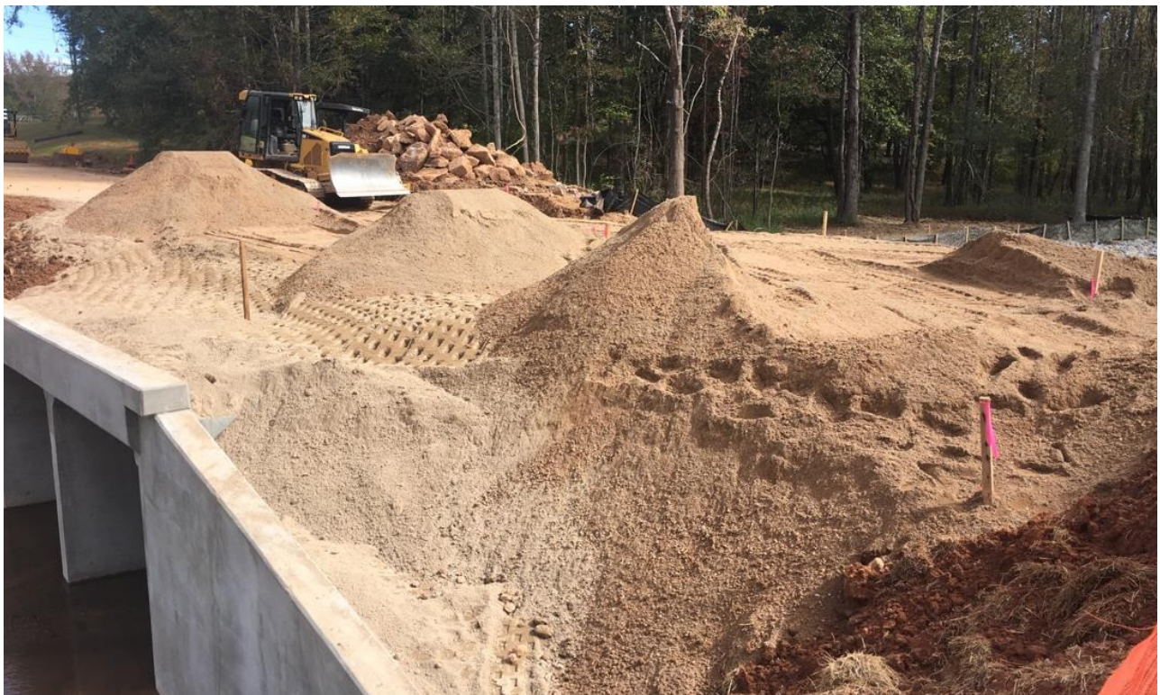
Photo 2: Backfill, compaction and grading are in progress. (11/01/2017)
