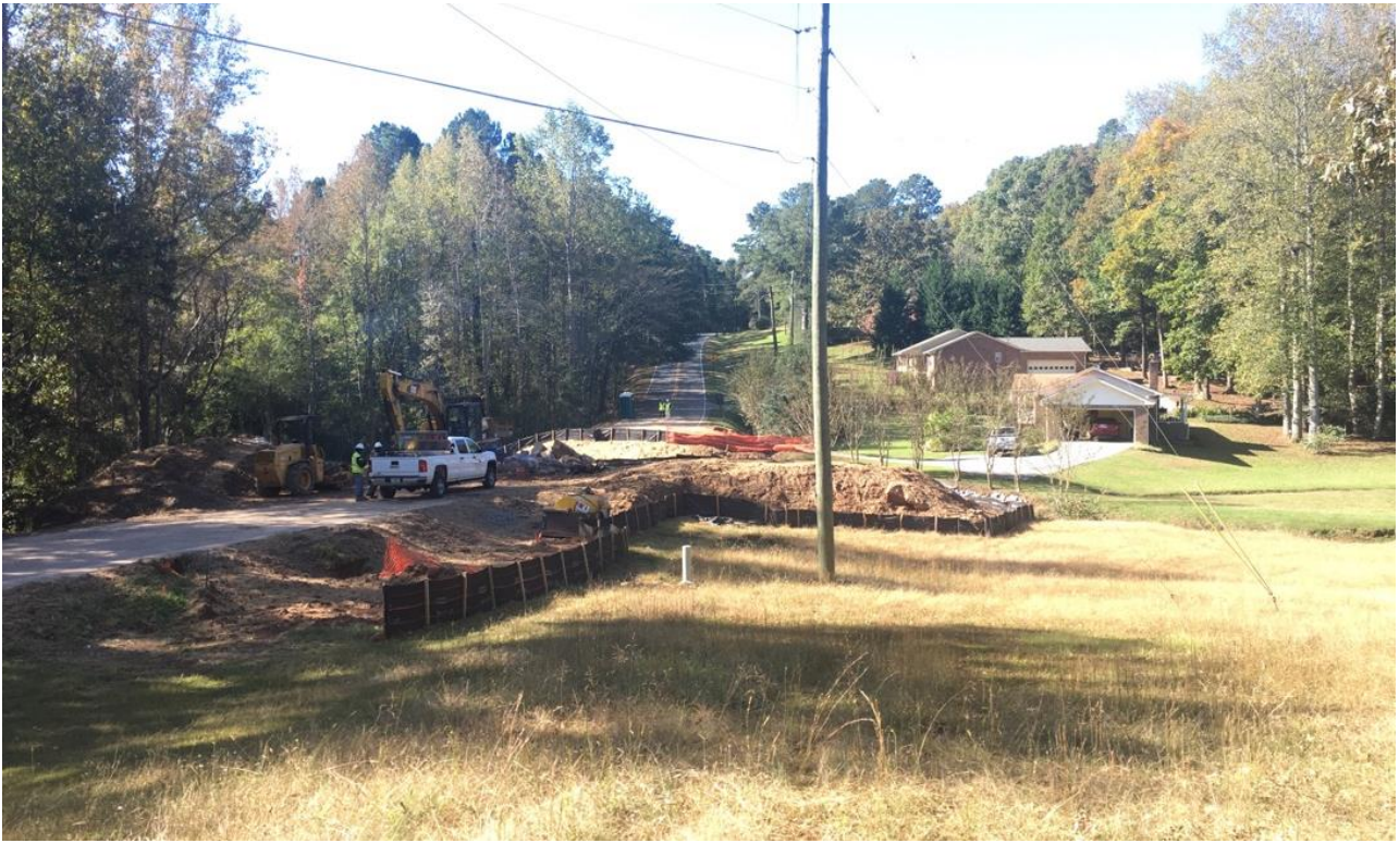
Photo 1: Field measurements are underway for shoulder grading and guardrail locations. (10/25/17)
