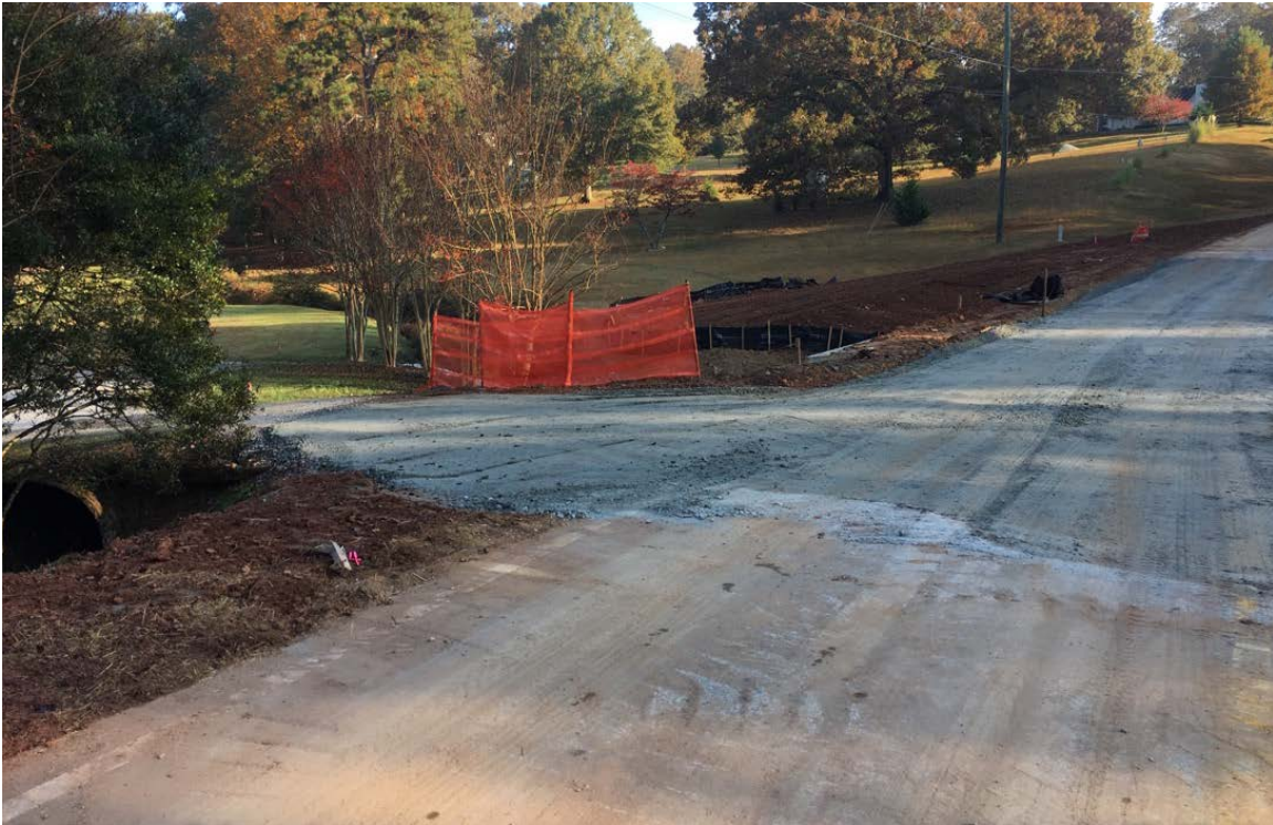
Photo 1: Roadway continues to be prepped for future paving. (11/06/2017)
