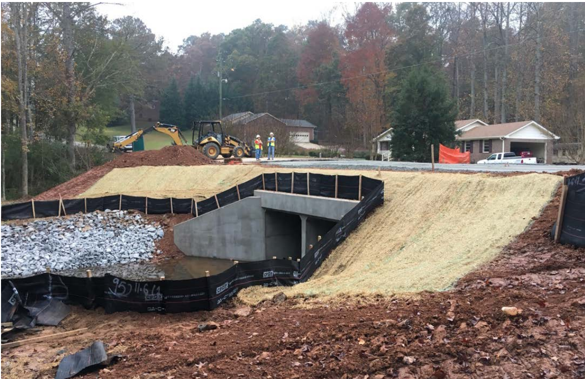
Photo 2: Soil stabilization has been placed along the south side of the road. (11/07/2017)
