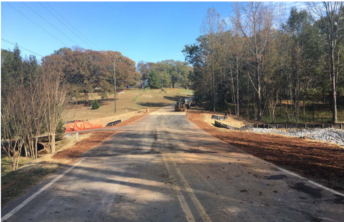
Photo 2: Additional fill has been placed and graded on the shoulder along the newly paved road section. The shoulder is prepped for guardrail installation. (11/14/2017)
