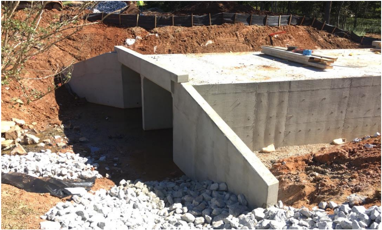
Photo 1: Culvert construction is now 100% complete (north side view).
