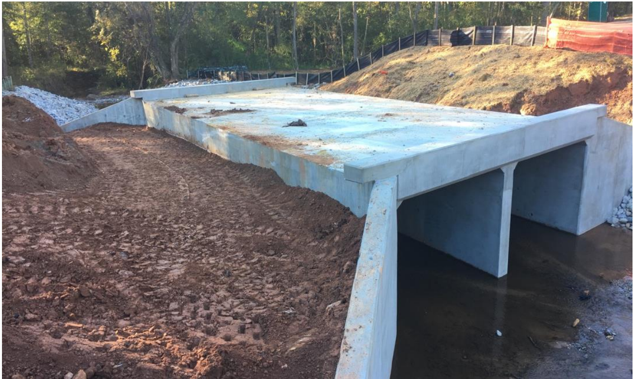
Photo 1: Back fill has been placed and compacted at the culvert. (10/27/17)
