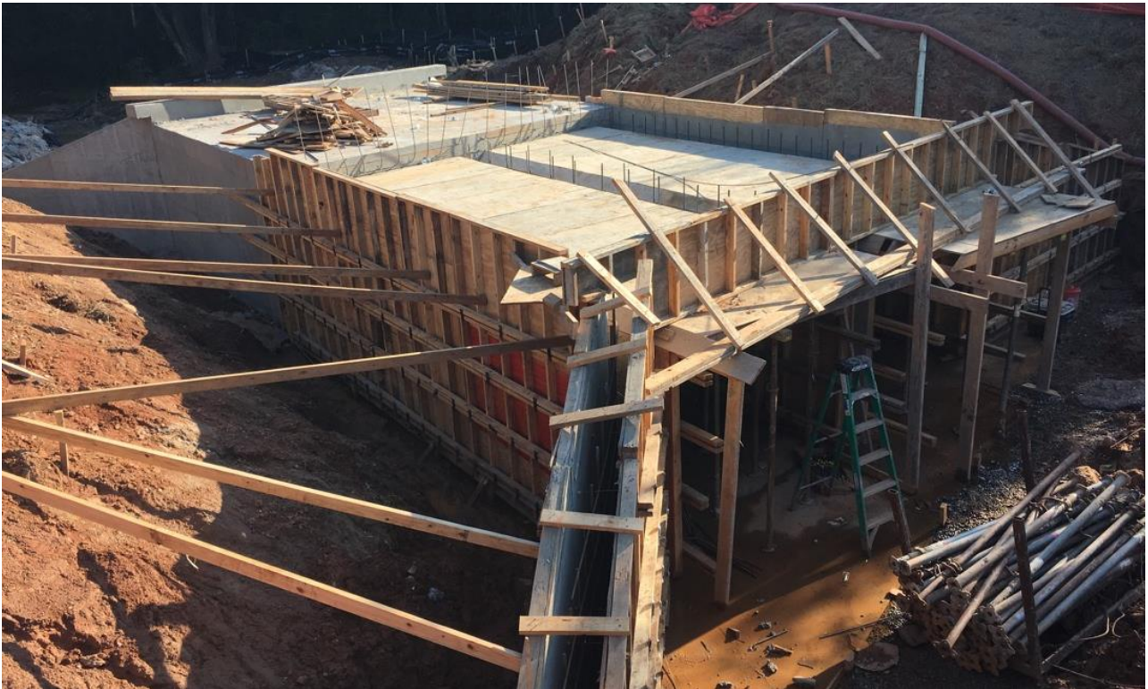
Photo 1: 2 nd Half of culvert: Rebar and forms have been installed.
