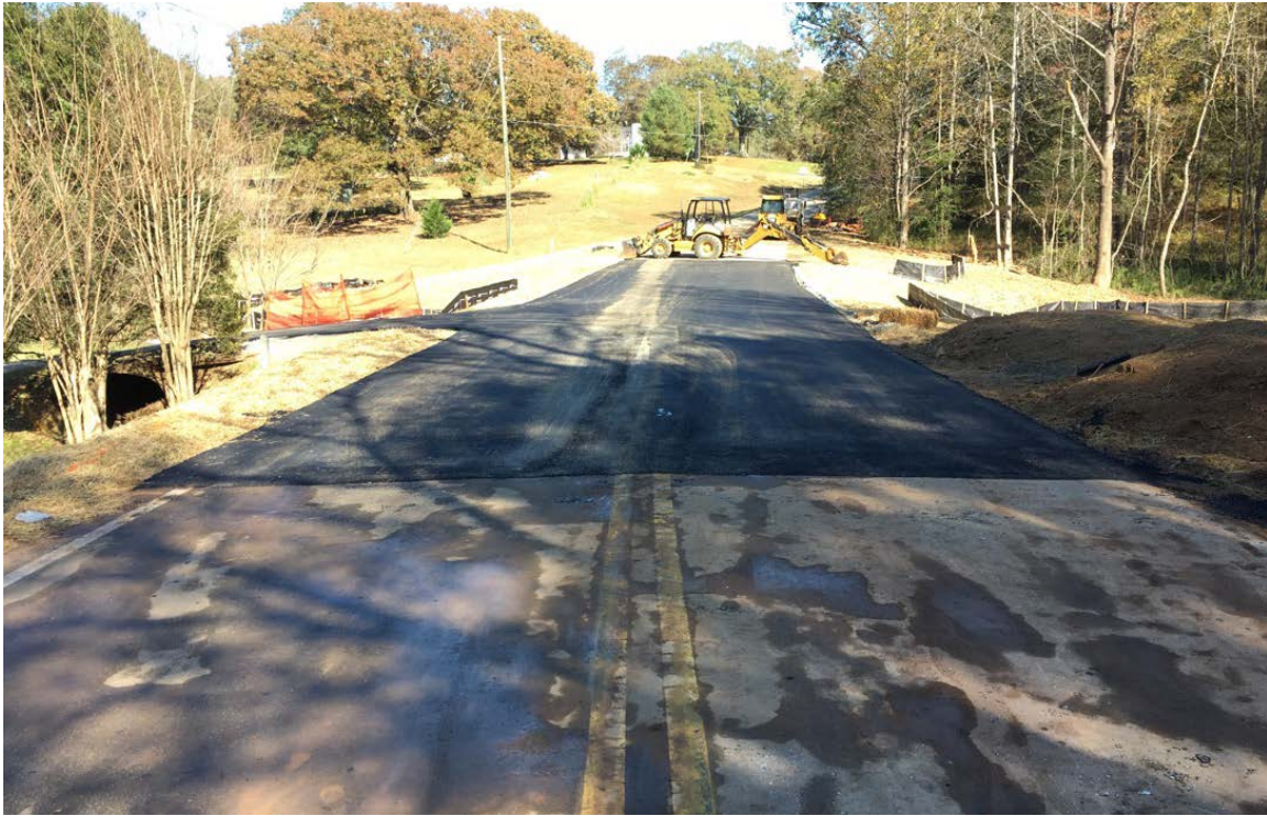
Photo 1: The road and residential driveway apron have been paved. (11/13/2017)
