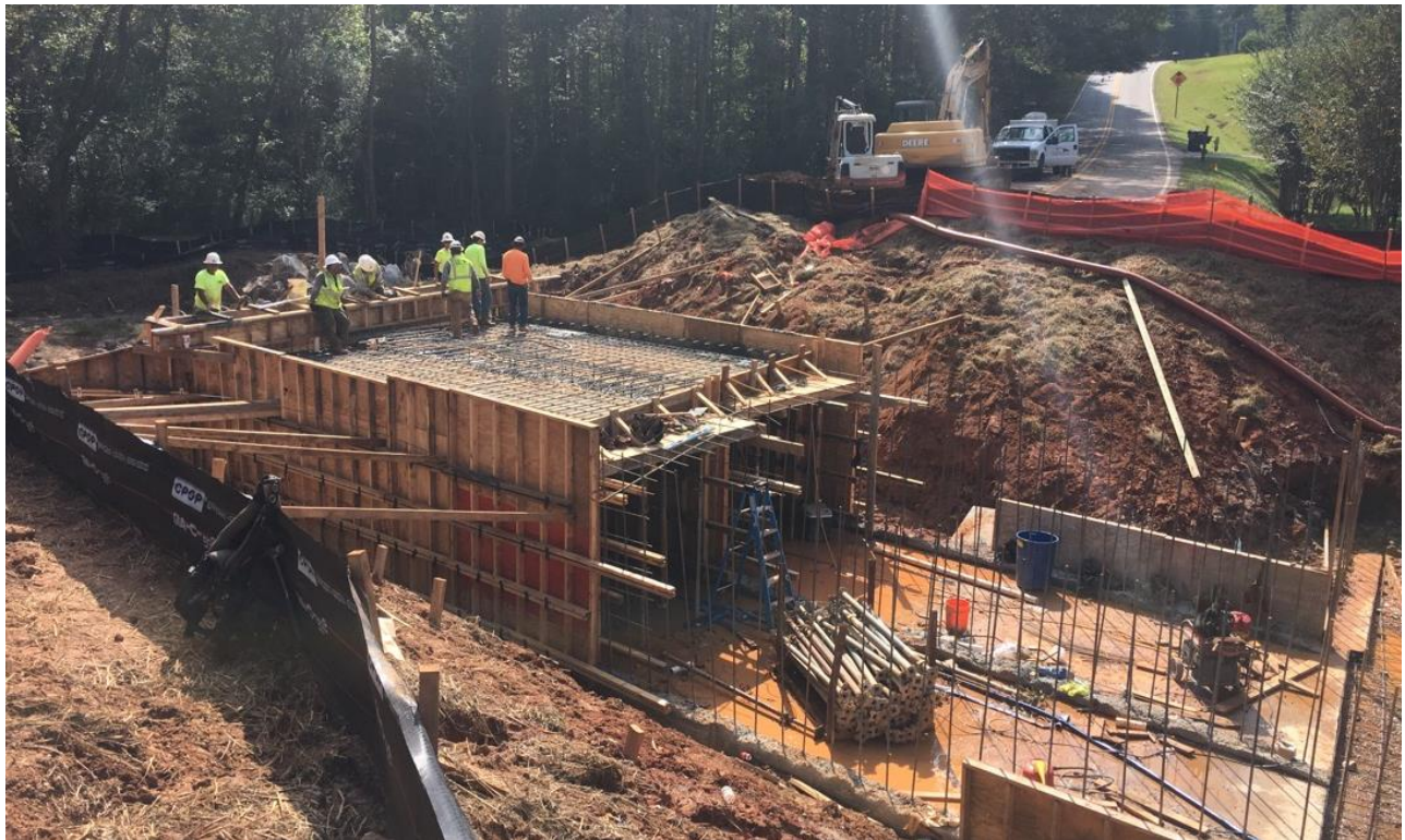
Photo 2: A concrete vibrator is being used for compaction in the walls.
