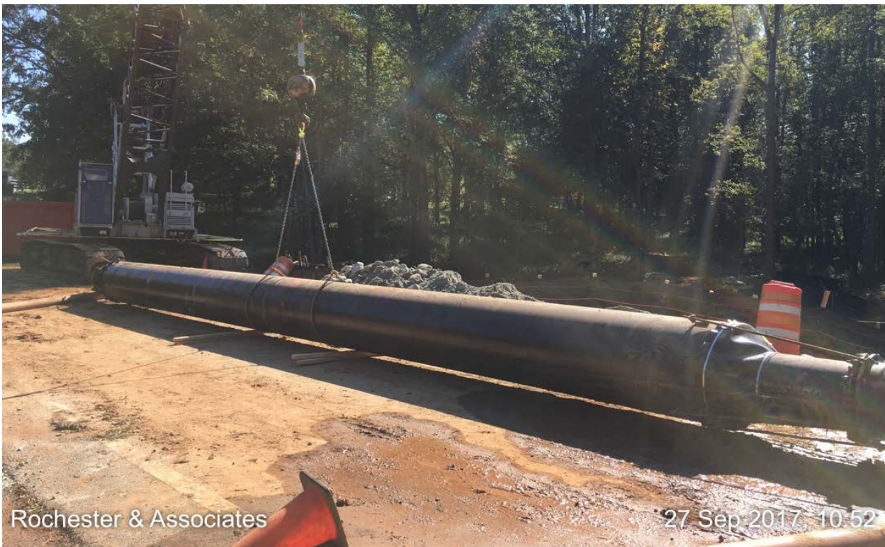
Photo 2: Culvert replacement design requires water line relocation. New water line (pictured above) is being installed.
